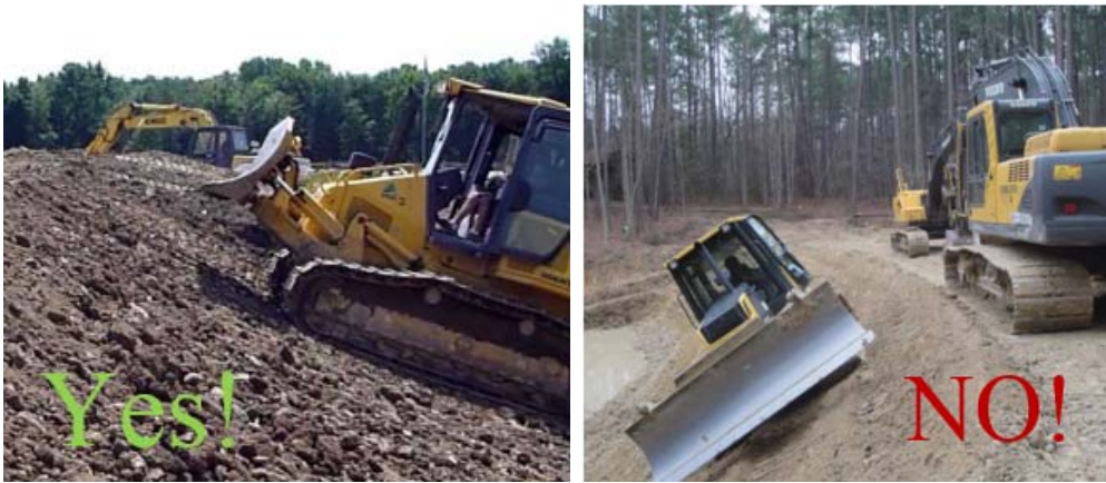
Figure 37. Proper and improper method for tracking slopes.
