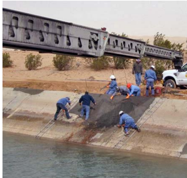
Figure 13. Replacing individual panels.
