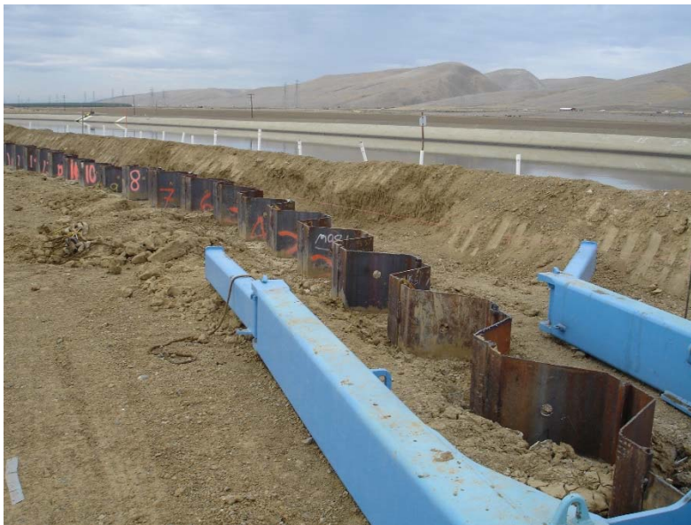
Figure 16. Sheet pile cutoff wall.
