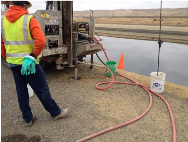
Figure 17. Grouting from the embankment crest.
