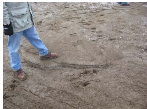
Figure 34. Surface erosion investigations.
