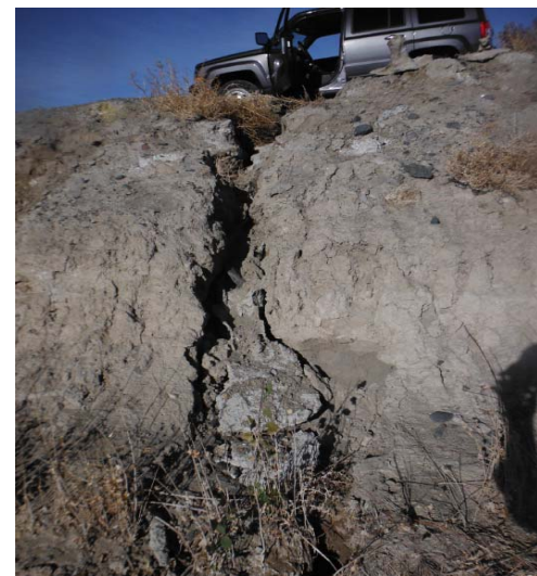
Figure 33. Examples of surface erosion.
