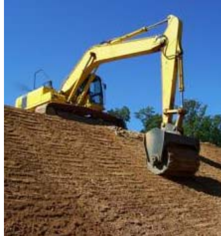
Figure 36. Repairing slope with an excavator attachment
