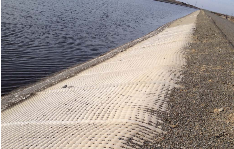
Figure 12. Example of a grouted mattress lining repair.
