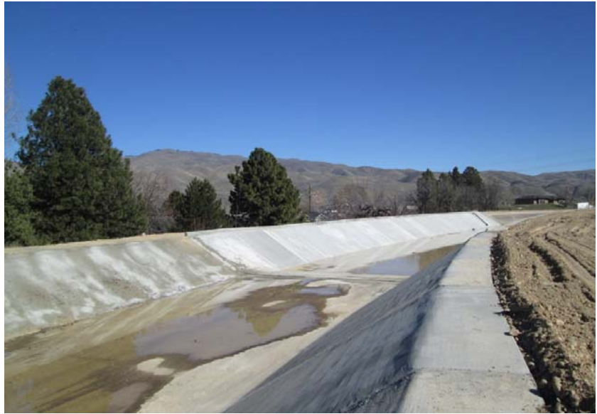
Figure 14. Completed concrete relined section of a canal.
