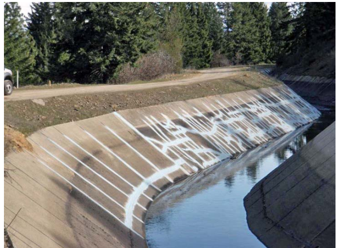
Figure 10. Example of crack and joint sealing.
