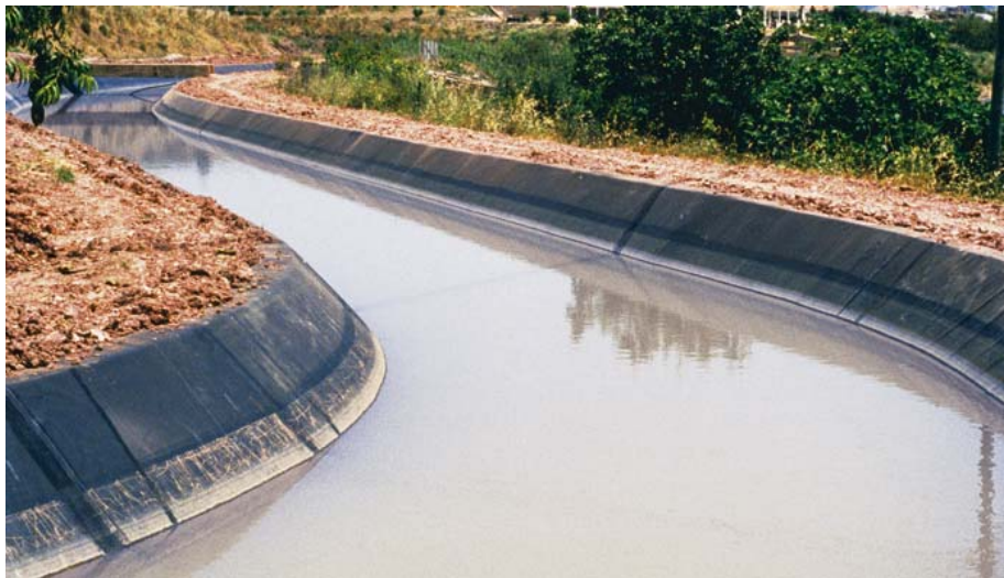
Figure 11. Example of geomembrane placed over a distressed concrete lining.
