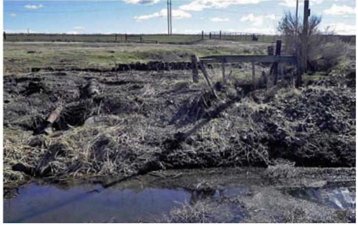
**Figure 2.** With the vegetation removed, miscellaneous pipes, fencing, and embankment distress emerges.
