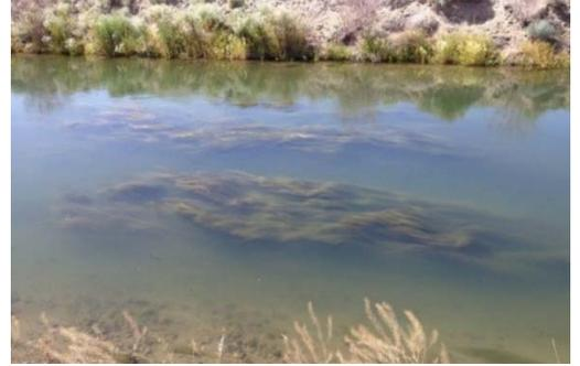
**Figure 7. Aquatic weeds impeding flow in a canal.**
