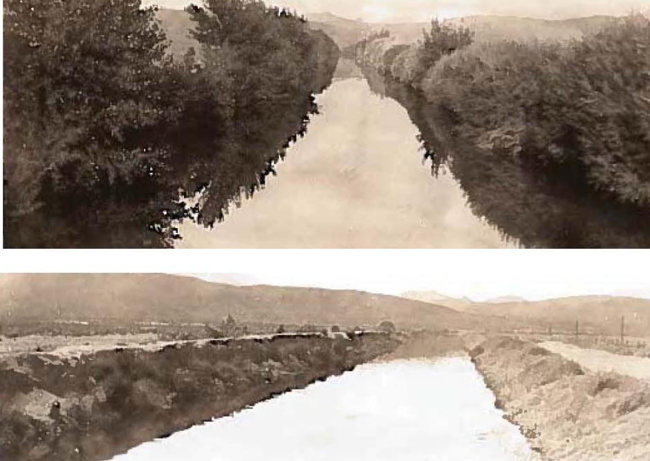
**Figure 14. Photos showing canal prism before and after vegetation removal. Note the disturbance to the canal embankment.**
