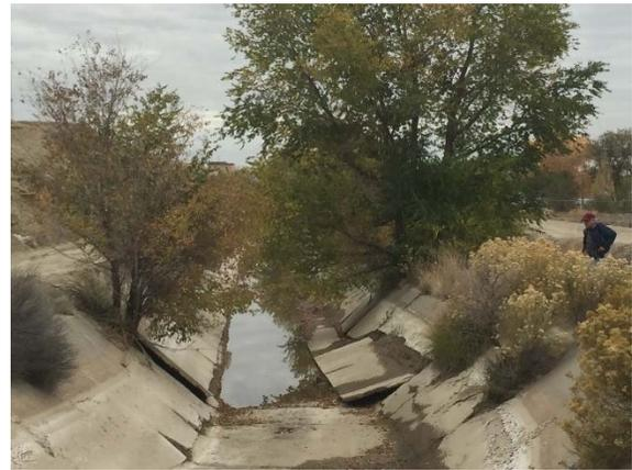
**Figure 3.** Extensive damage from trees on a concrete-lined canal.
