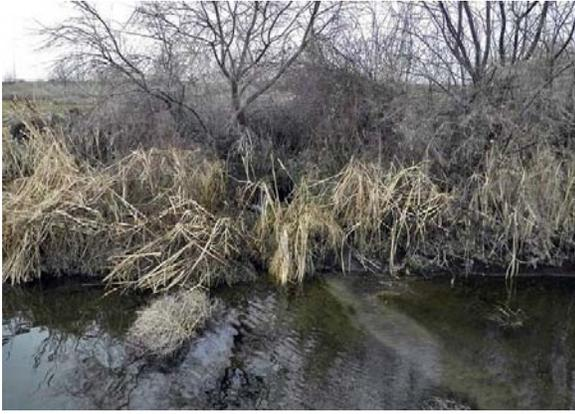
**Figure 1.** The vegetation in this canal prism is overgrown.
