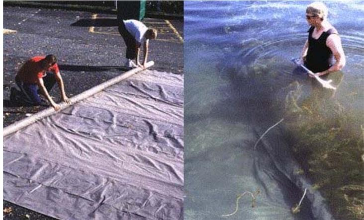
Figure 30. Installing bottom barriers.
